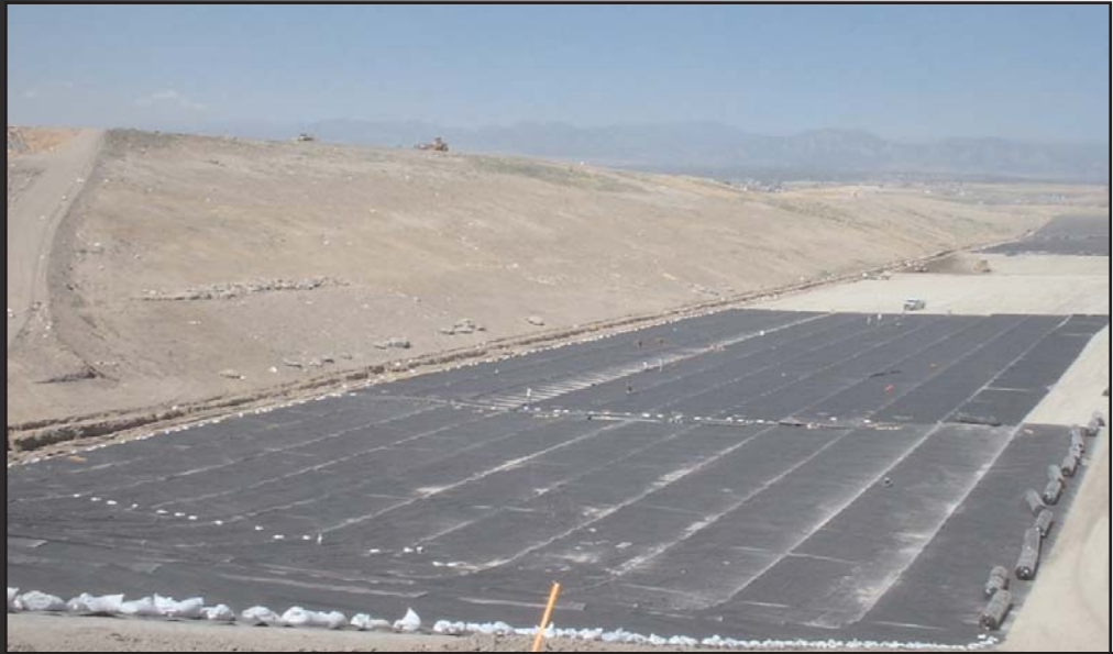
FRONT RANGE LANDFILL --- ERIE, CO --- 510,000 SF --- 60 MIL TEXTURED HDPE
