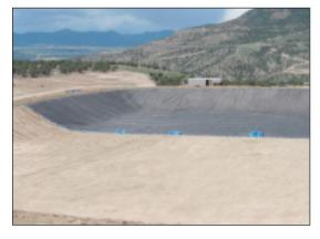
Supportive materials are often necessary for containment that are reliable and extremely safe for the environment. These specialty materials like GCLs, Geocomposites and Geotextiles add peace of mind and confidence to the ability of a complete system.
