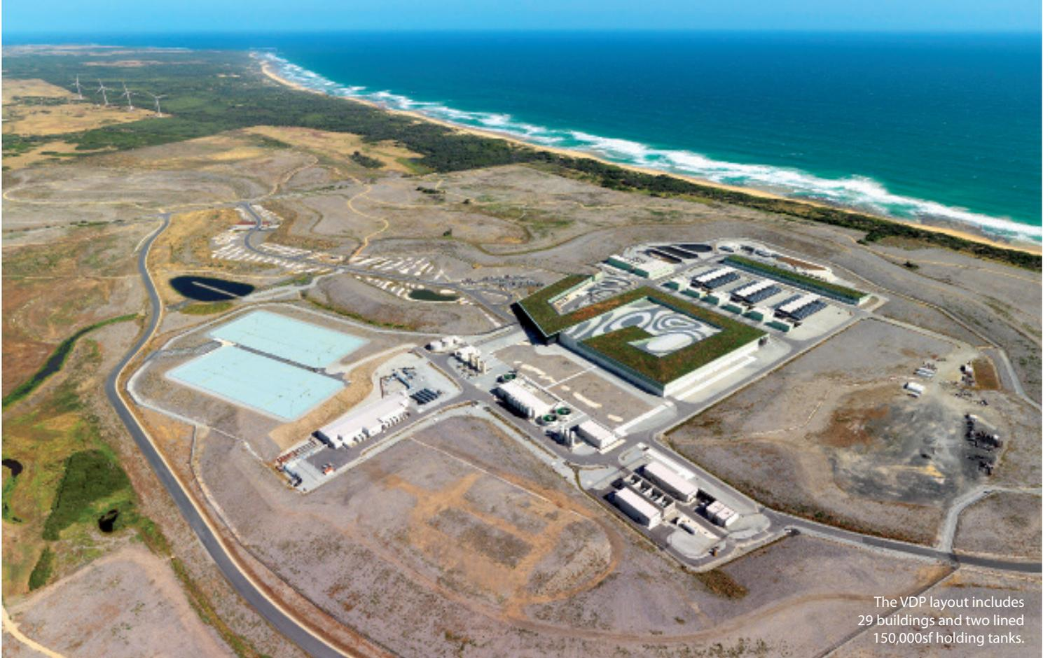
The VDP layout includes 29 buildings and two lined 150,000sf holding tanks.
