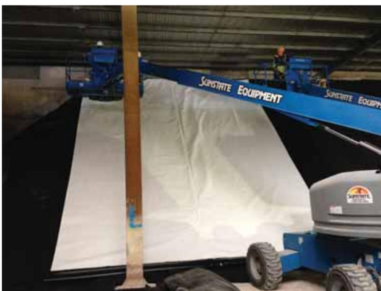
PHOTOS 3 AND 4 Aerial manlift—extrusion patching from tray.
