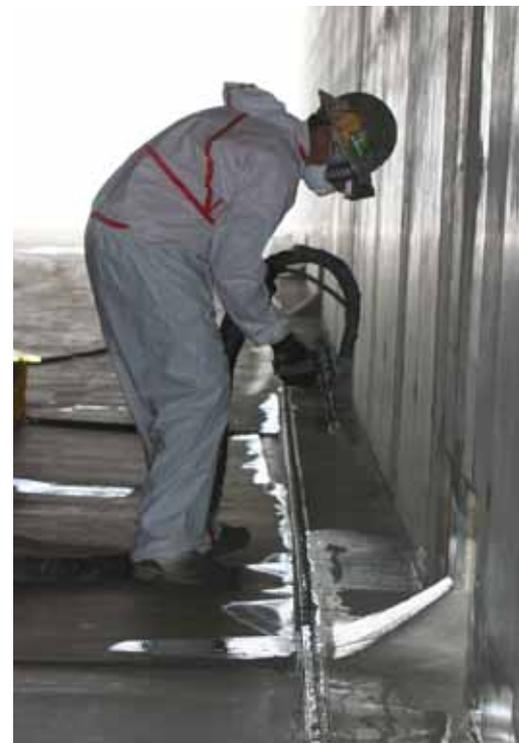
PHOTO 2 Coating is applied along the baffle wall.
