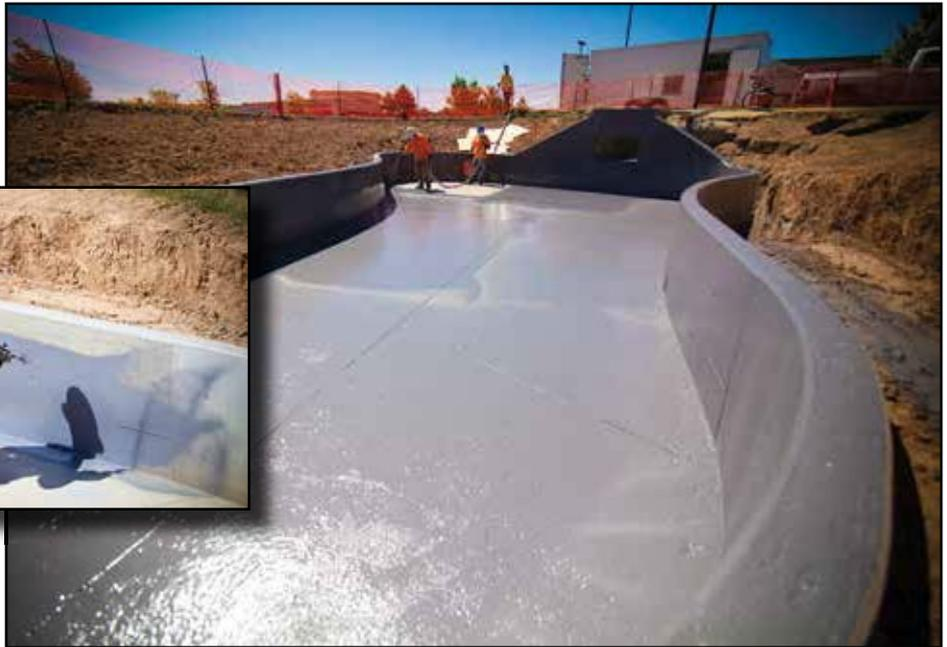
**An underdrain was added to this rain garden, as well as infiltration and growing media, and native plants. Inset: The spray-applied membrane decrease stormwater runoff volume as the garden removes pollutants in runoff through natural vegetative processes.**
