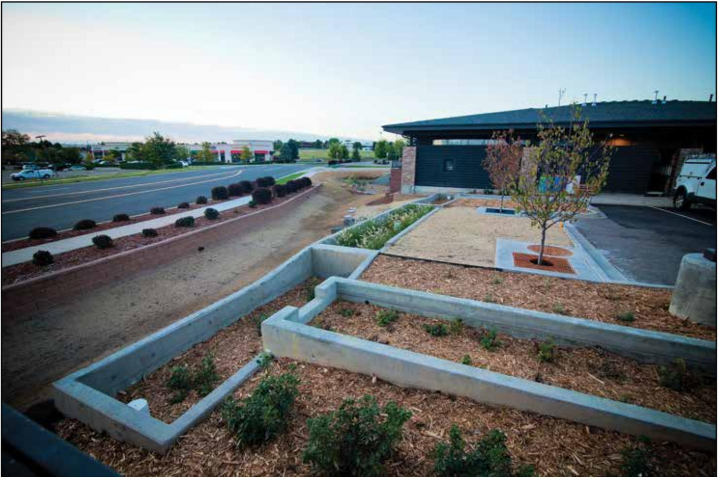
**The site efficiently incorporates a range of readily available green technologies, including the bio-mod units, two tree filters, a living wall, the bioswale, and the SEMSWA rain garden. Collectively, these systems form a “treatment train” to treat runoff.**
